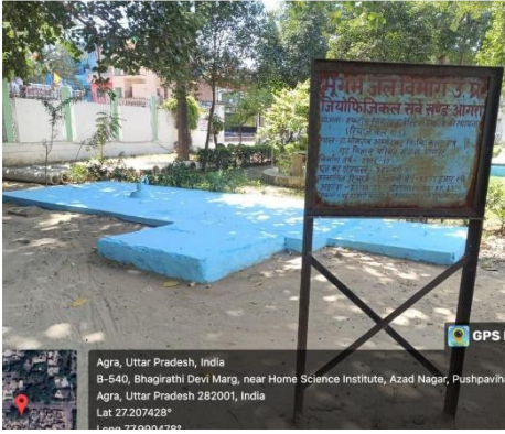
Rainwater harvesting pit
