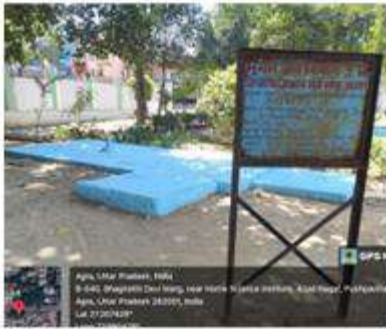
Rainwater harvesting pit
